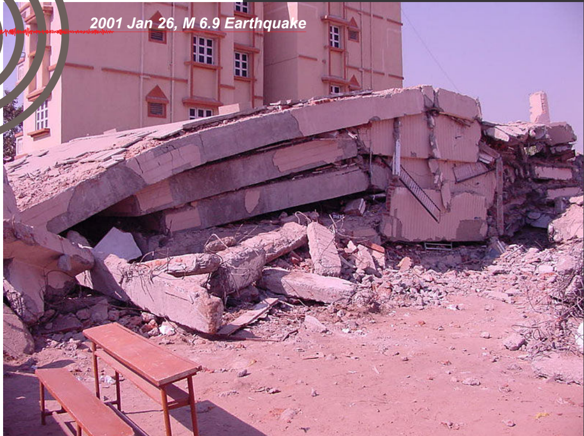
Pancake collapse of 4-storey L-shaped RC framed school building in Ahmedabad city, situated more than 245 kms away from the earthquake epicentre. The building collapse killed 32 children. The building had a weak structural system.
